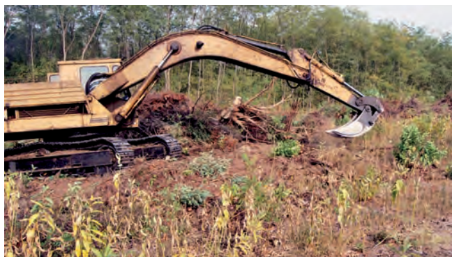
Fig. 3. Stumping excavator with fork attachment. (Photo: A. Csór)
