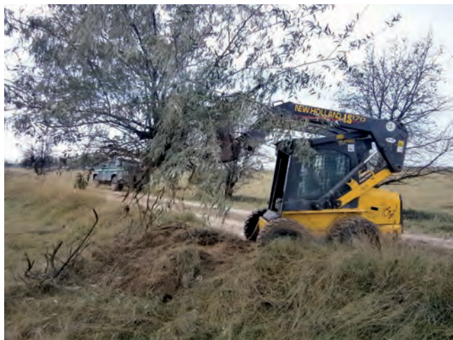
Fig. 3. Front-end loader tractor extracting a Russian olive with the root structure. (Photo: Cs. Vadász)
