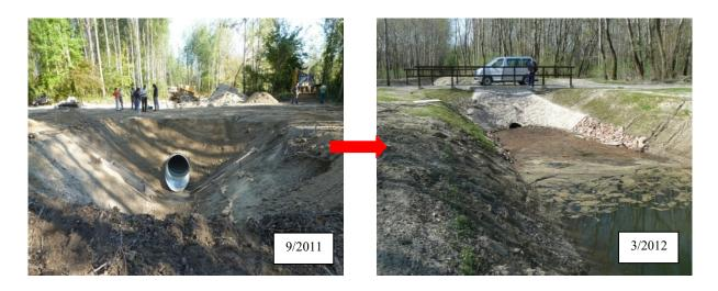
At the forestry road crossing the TUBOSIDER culvert was built with its concrete and wooden elements. In the downstream side a water level height measuring point was established. The culvert is prevented from the floating debris with iron rods on both ends. After the field works the final geometry was measured by geodetic survey. The realization plan was created by Irányszög Bt. Number: 2011/V/03.
