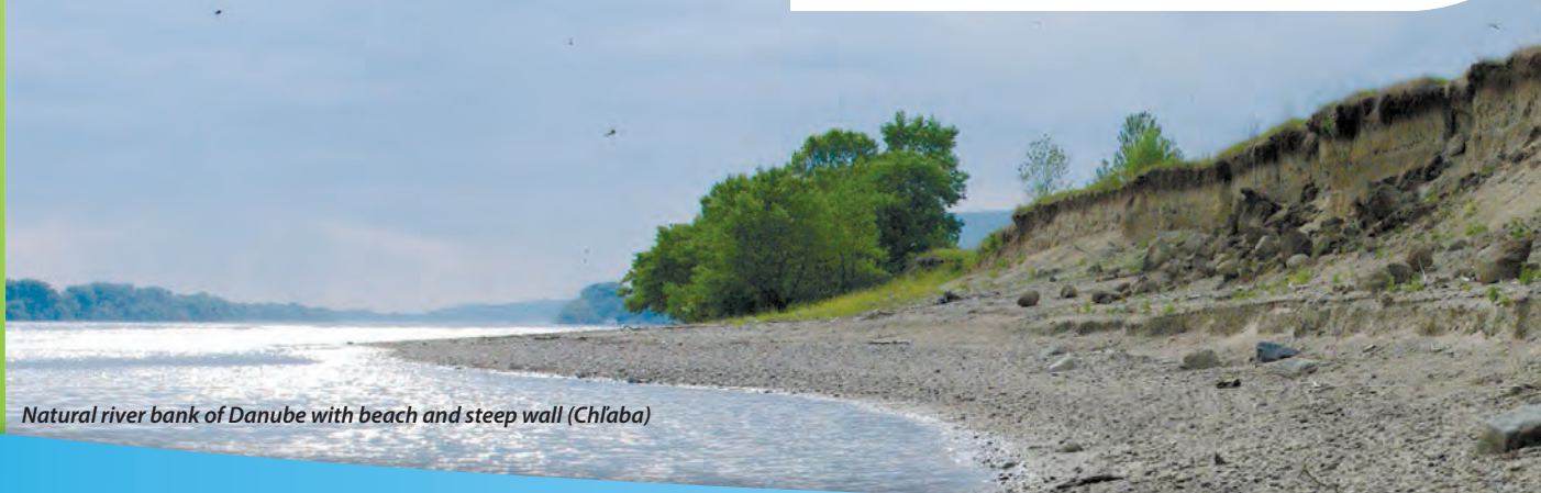
Restoration of natural river bank (Zlatná na Ostrove)
