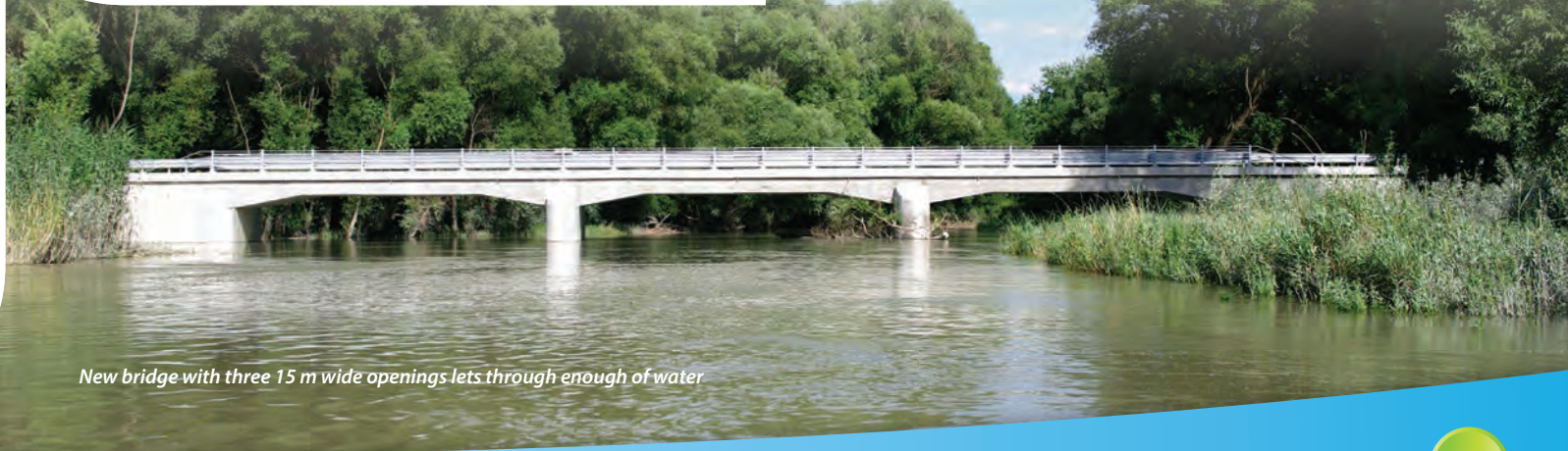
Former culvert through the river branch had the size of 2x2 m
