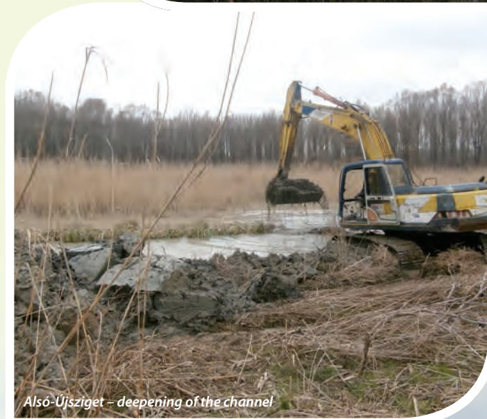
Alsó-Újsziget – preparation of the restoration
